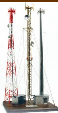
Self Support , Guyed , Mono-Pole Towers
